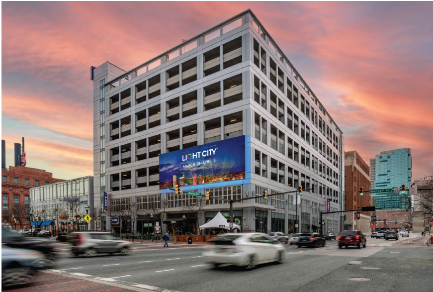
124 Market Place (NE Corner)
